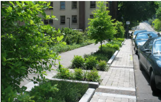
Bioretention Planting Strip | City of Portland, OR
