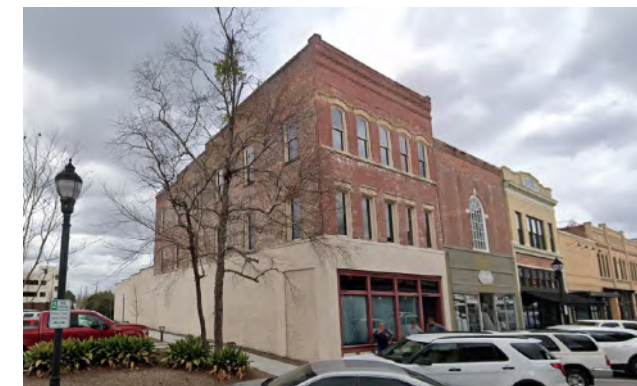
127 West Evans Street Renovation After | Google Earth
