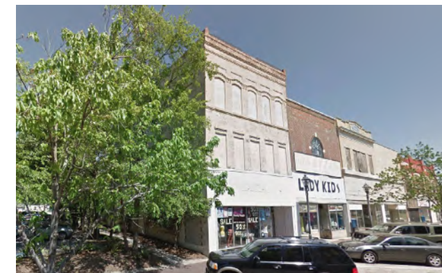
127 West Evans Street Renovation Before | Google Earth
