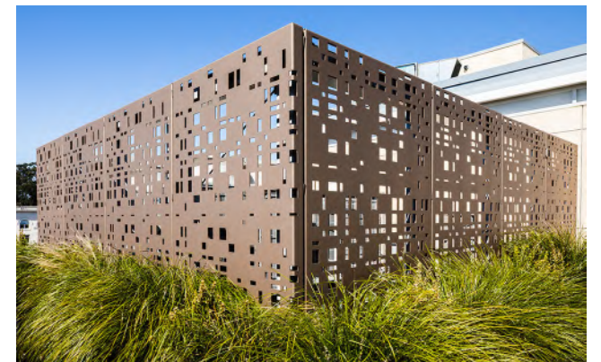
Mechanical Equipment Screening | BOK Modern
