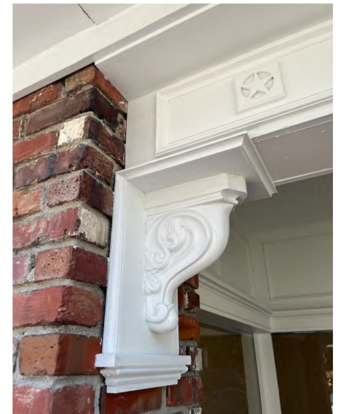
Preserved Cornice On A Downtown Florence Storefront
