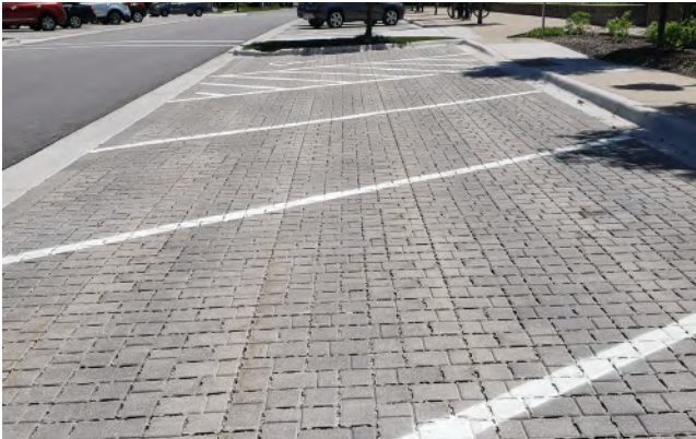
Pervious Parking Paving | City of Warrenville, Illinois
