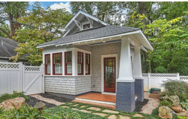
Complementary Accessory Structure | Hopedale Builders
