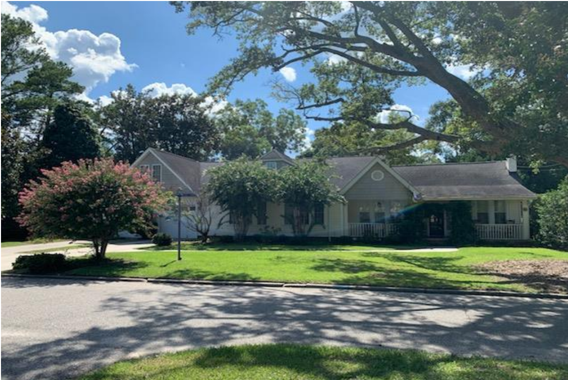
Front of 311 South Franklin Drive
