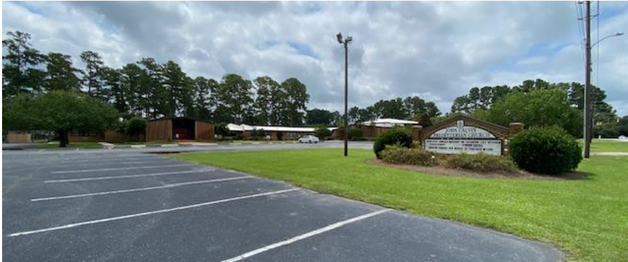
The western half of the parcel with the church building along Marsh Avenue to remain CA.
