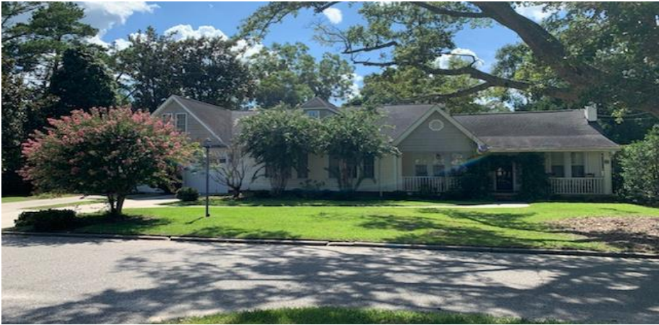
Front of 311 South Franklin Drive
