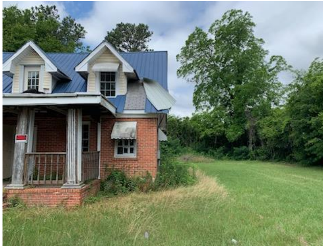
621 South Church Street – Home Encroaching 2.1'
