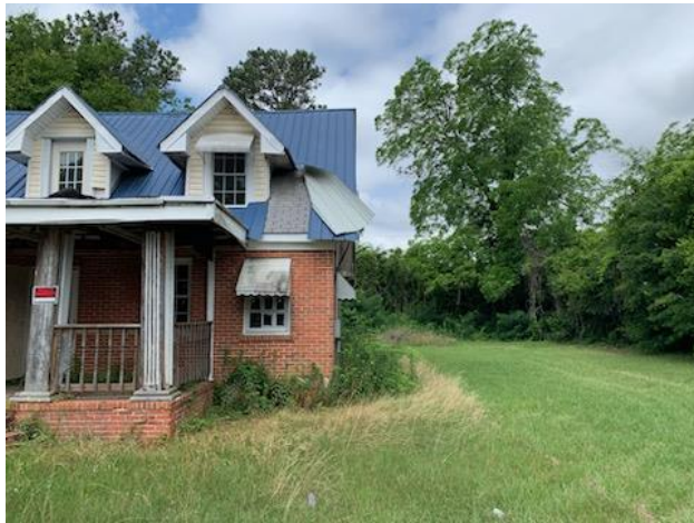
621 South Church Street – Home Encroaching 2.1'
