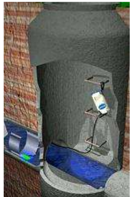
Figure 1: Typical Flow Monitor Installation in a Sewer Manhole
