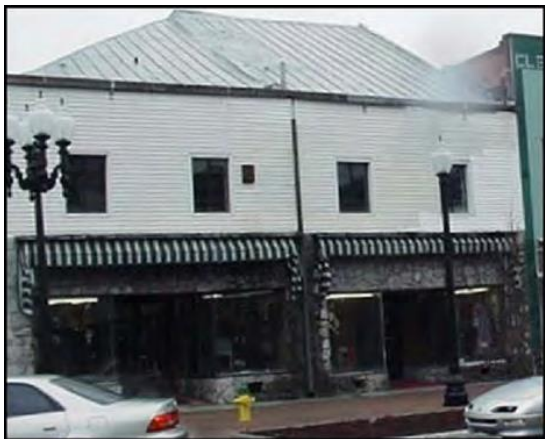
This historic commercial building has been inappropriately renovated. The use of siding on the second level and formstone "fieldstone" on the first level hides what might have been an attractive building. In addition, the size and proportions of the windows on the second floor are out of scale with the building.
