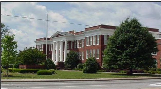
Buildings such as the new library and the National Register Poynor School help define the parameters for architecture and site design in the Arts & Cultural District.
