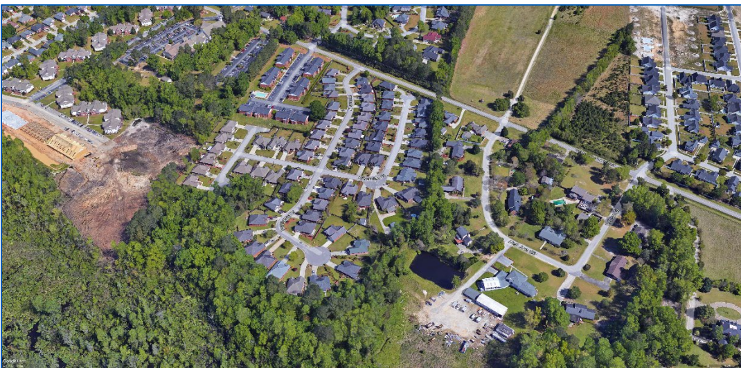
Inverness Estates (at center of image) along 3 rd Loop Road in south Florence.
