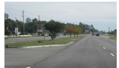
View of East Palmetto Street, looking eastward as it approaches the airport. The street cross section includes a landscaped median with turning lanes. Enhanced landscaping and minor repairs would greatly improve the appearance of this roadway.
